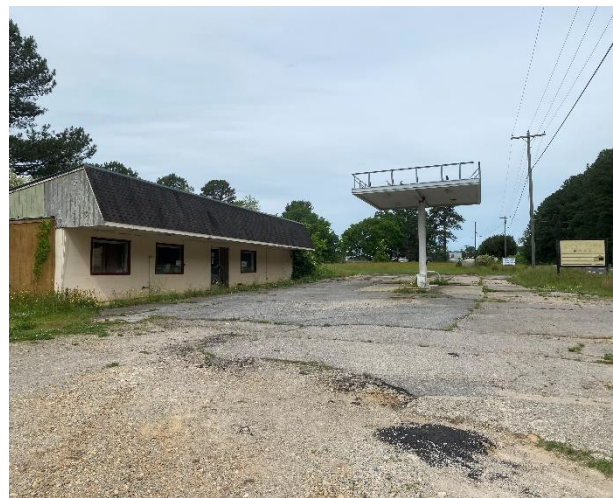
Figure 6: Eaton's Ferry Grocery and Grill site (~1249 ft from petitioned parcel)
