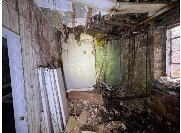
Photo #48 – Collapsed Ceiling
