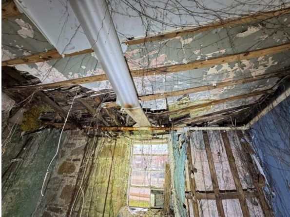
Photo #47 – Collapsed Ceiling
