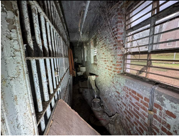
Photo #79 – Rear Jail Cell
