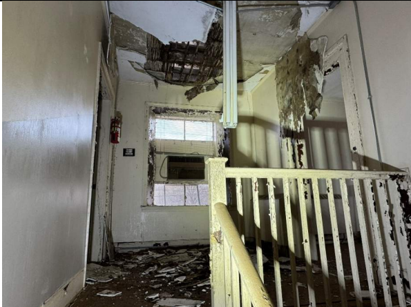
Photo #47 – Collapsed Ceiling
