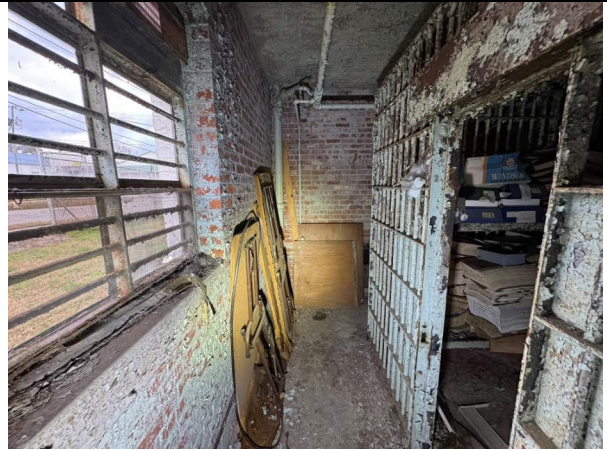
Photo #80 – Rear Jail Cell
