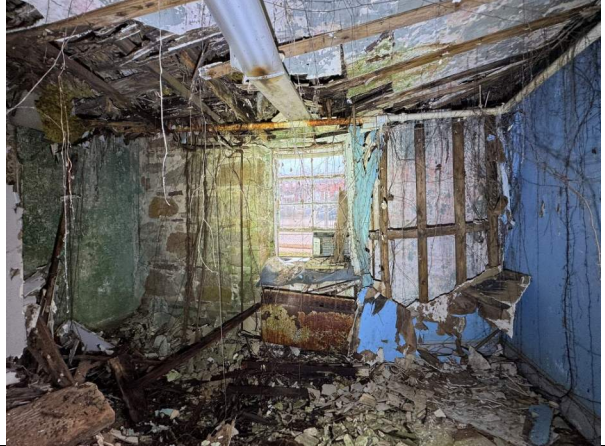
Photo #46 – Collapsed Ceiling & Floor
