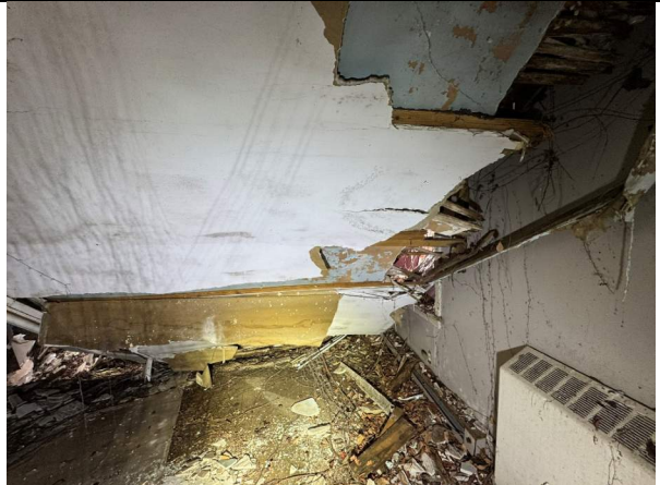
Photo #48 – Collapsed Ceiling
